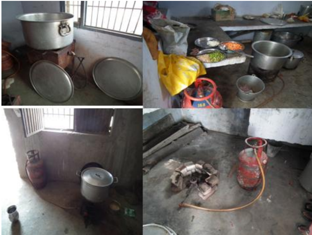
NON STANDARDISED GAS REGULATORS AND GAS PIPES
